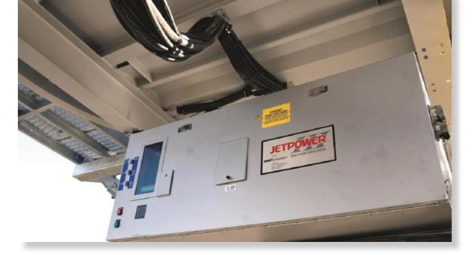
Jetpower® III The Jetpower\* III uses pulse width modulation technology to convert energy to 400 Hz ground power for airport applications. The unit can be mounted on the passenger boarding bridge or on a cart for greater mobility. Jetpower® III inverters utilize maintenance free, state-of-the-art technology.
